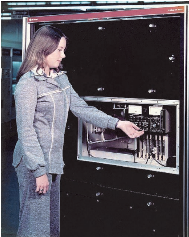
The original 10 KW PA Engineering Unit. This photo was taken to advertise the "built-in-test" and maintenance features of the new Power Amplifiers
